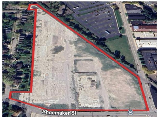
Aerial: After Demolition
