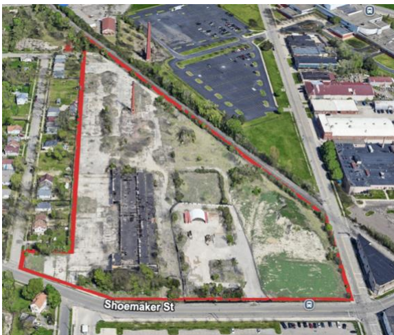
Aerial: Before Demolition
