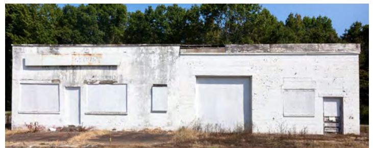
Former Auto Repair Shop, Washington
