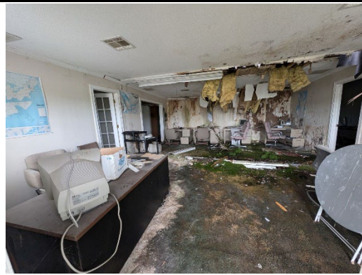
Shed Interior – Water Damage
