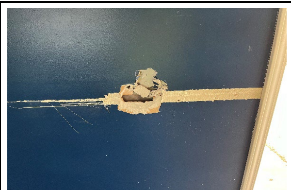
AS 3-1 Drywall With Joint Compound
