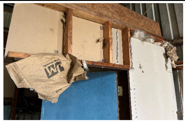
AS 4-1 Rolled Insulation
